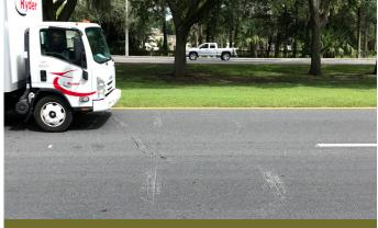
Permanent count station are sites that feature infrastructure that has been installed into the roadway surface. 'Loops' replace the use of pneumatic tubes used in temporary stations. These subsurface loops are fixed and can be connected to a portable count computer or a permanent cabinet. These stations allow for basic counts, as well as the capability to determine vehicle class and speed.
